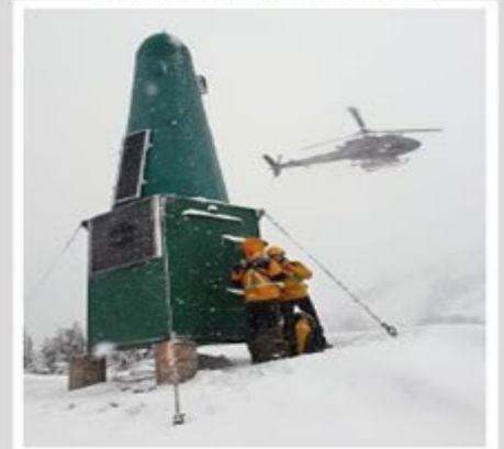
Mount Johnson Repeater
